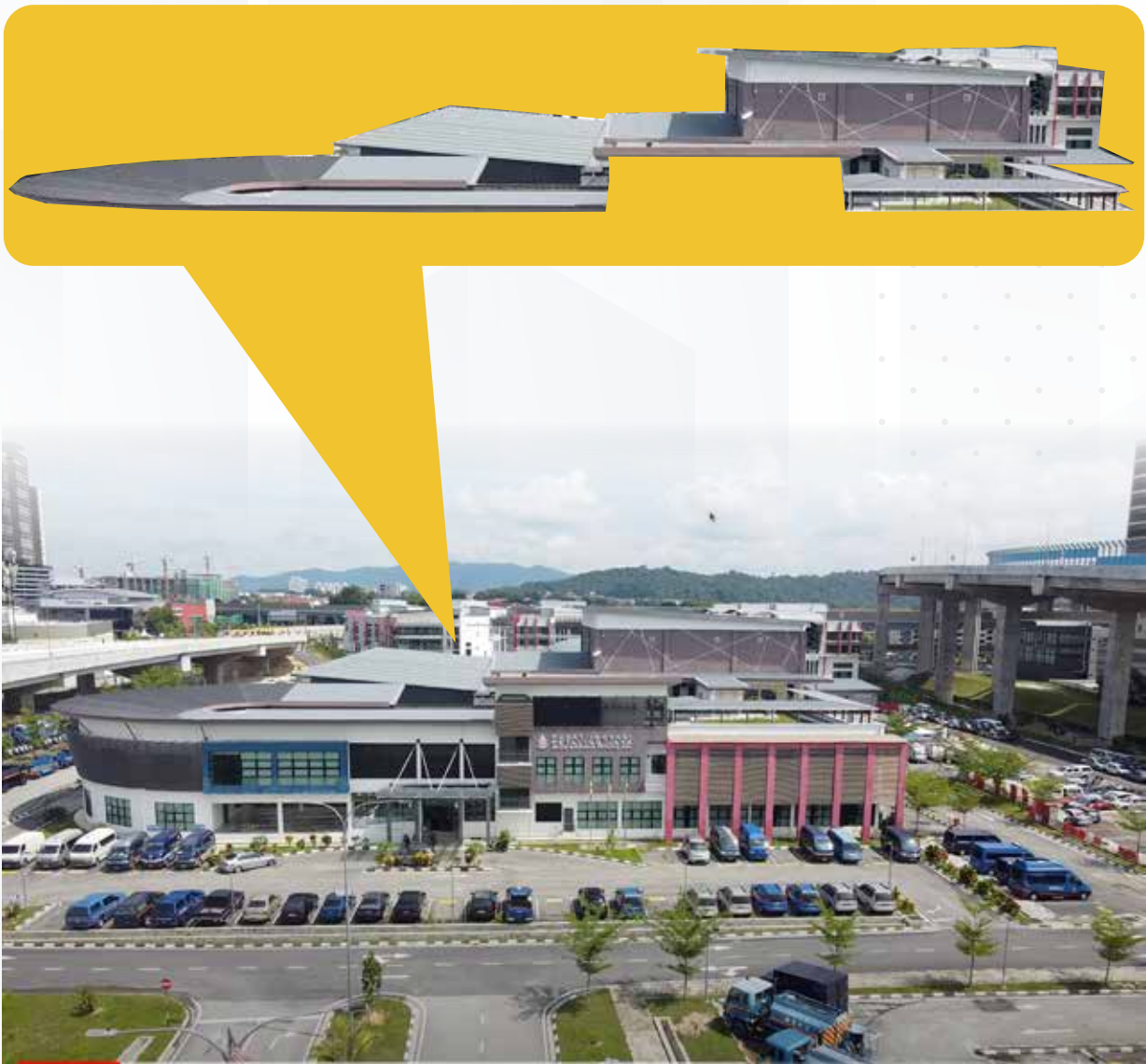
Installation rooftop Solar PV with ESCO Capacity = 250 kWp
